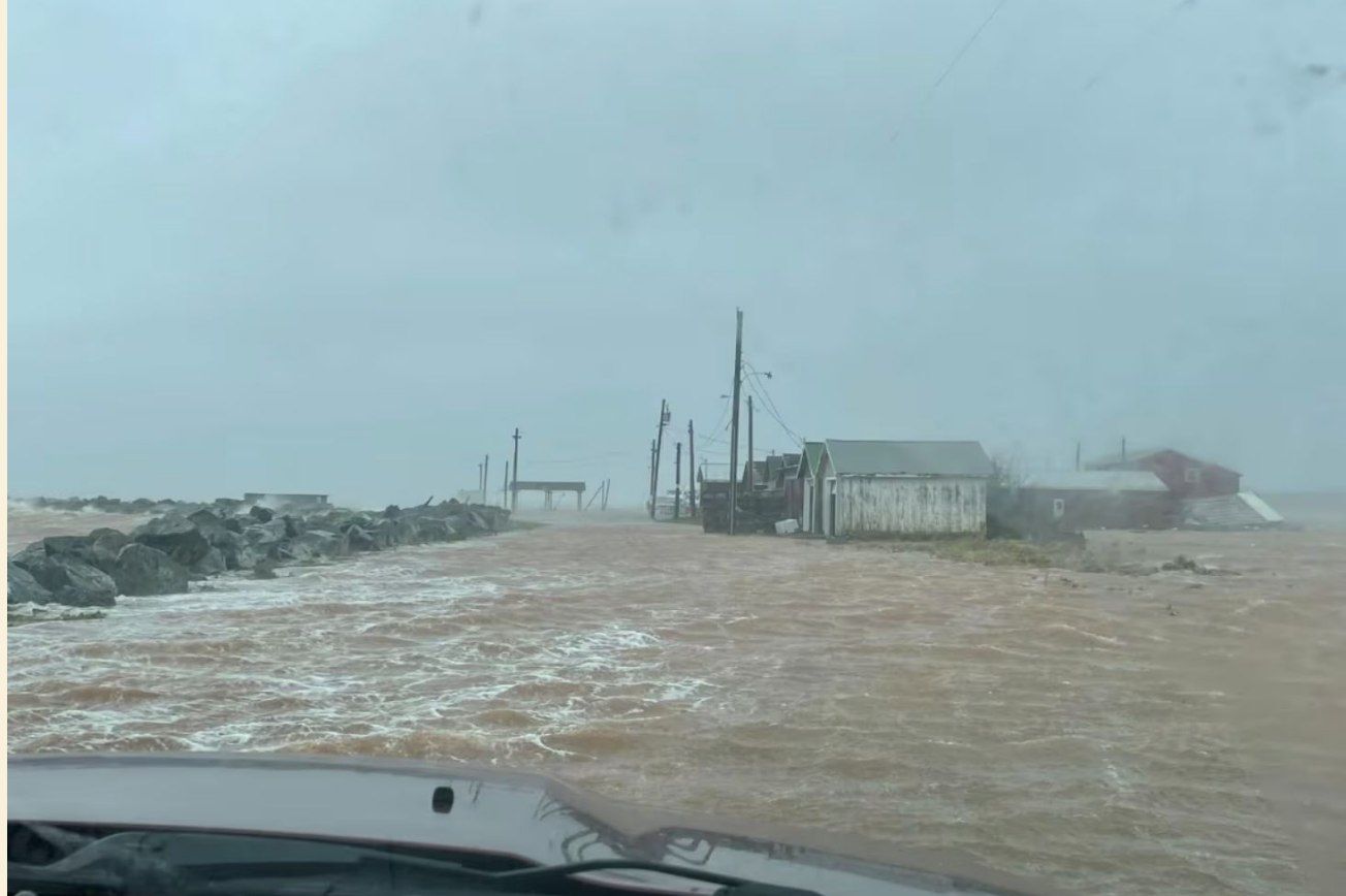
TRACADIE, PEI — A washed-out at Tracadie Wharf Sunday, Sept. 22, 2022 caused by hurricane Fiona. The storm washed out wharfs, tore roofs off of homes, overturned cars and buildings, felled power lines and many trees across the Island. (Devin Wolters/ CBC Online)
